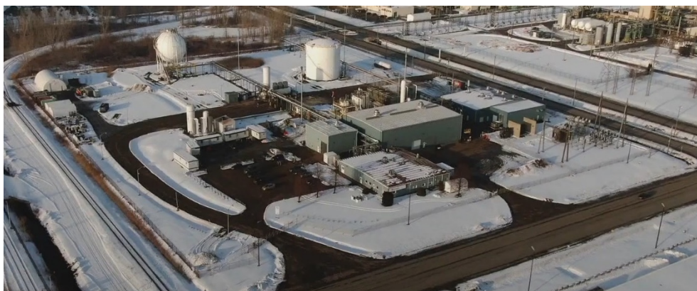
Figure 19: Industrial-scale proton exchange membrane electrolyser (20 MW & 3000 t/year – Becancur, Canada)
