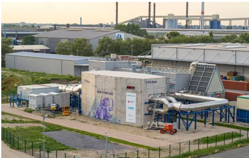
Figure 16: Electric thermal energy storage demonstration plant (130 MWh – Germany)
