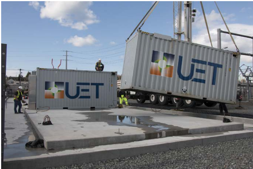
Figure 14: Vanadium redox flow batteries at commercial scale (2 MW/8 MWh – Seattle, USA)
