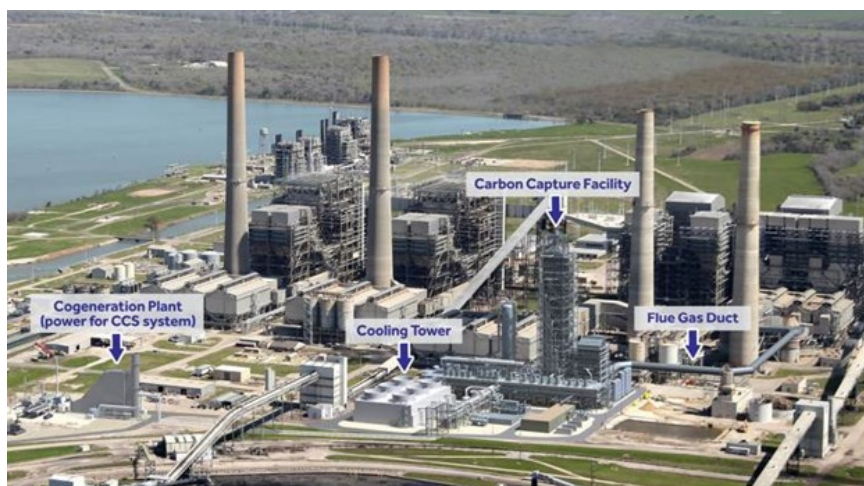
Figure 17: Post-combustion CCS at Petra Nova (240 MW – USA)
