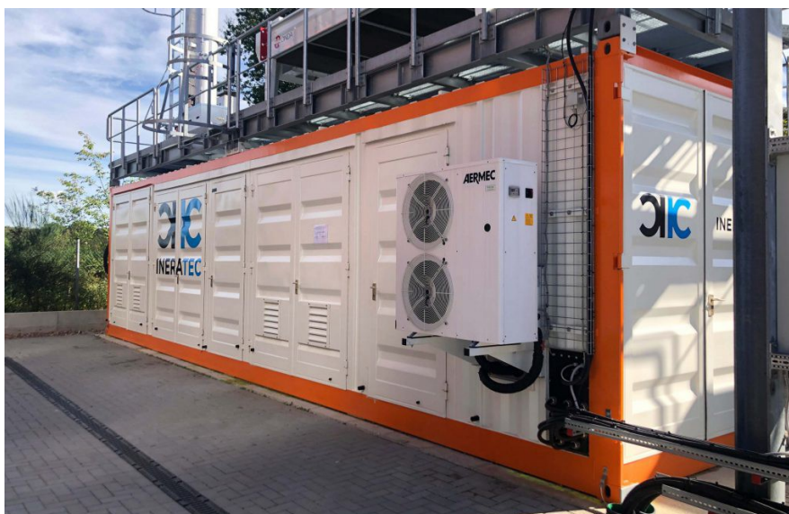
Figure 28: Existing Ineratec PtX plant (≈350 000 kg/year – Germany) 99
