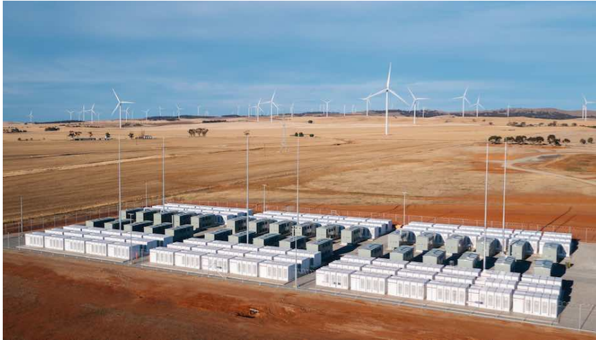
Figure 13: Utility-scale battery energy storage system used primarily for frequency regulation (and some energy arbitrage) at Hornsdale Power Reserve (100 MW/129 MWh – Australia)
